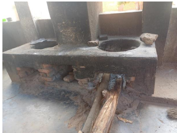
Rehabilitation of main student stove
