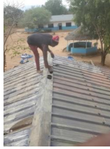
Fixing loose panels
