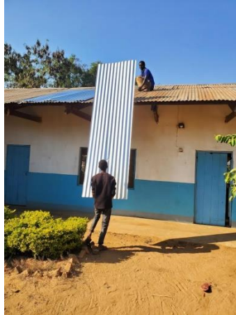
Replacing roof sheets
