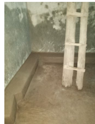
Internal plastering
