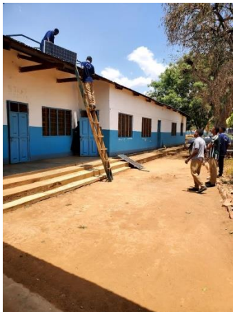
Replacing solar panels
