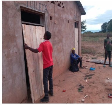
Fitting new doors
