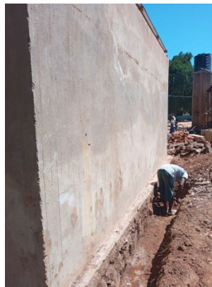
External plastering of the tank
