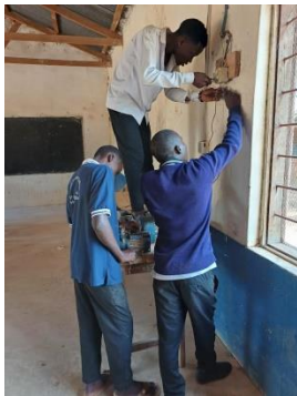
Practical electrical work
