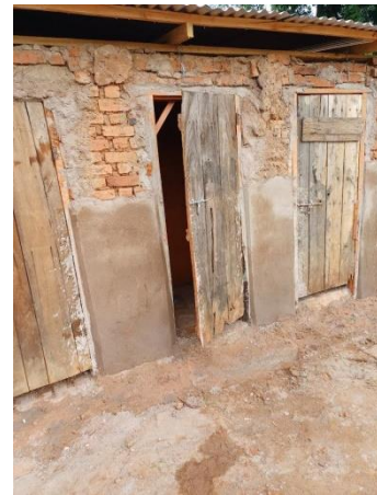
Toilet block before rehabilitation
