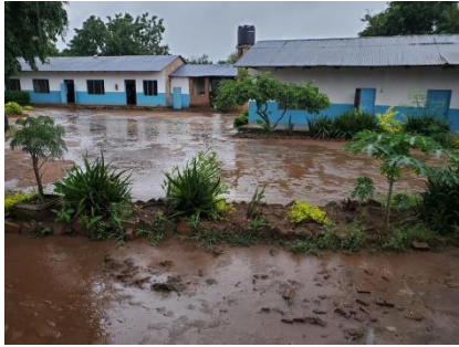
Flooding around the college buildings
