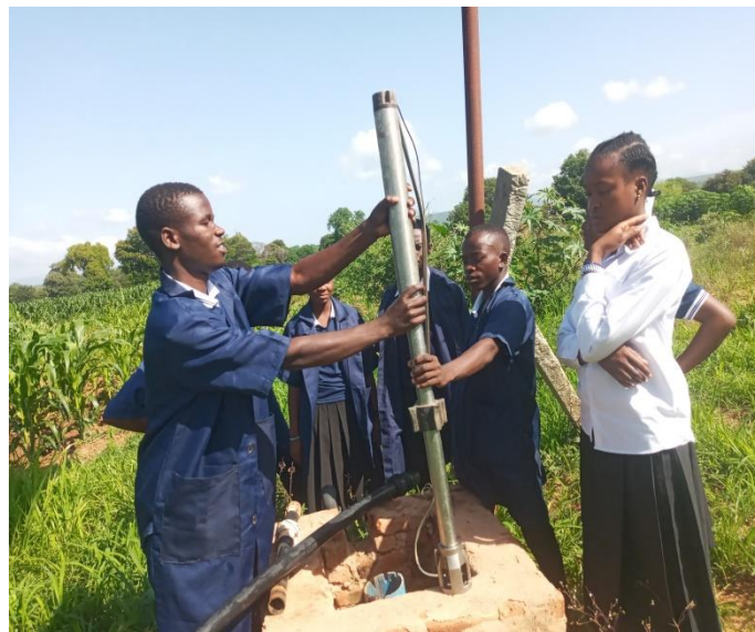
Electrical students installing the new solar pump
