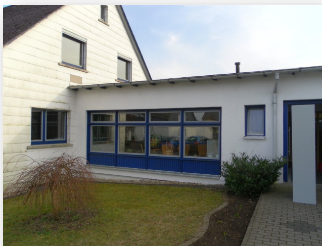
The CP house in Stahlhofen am Wiesensee, Germany.
