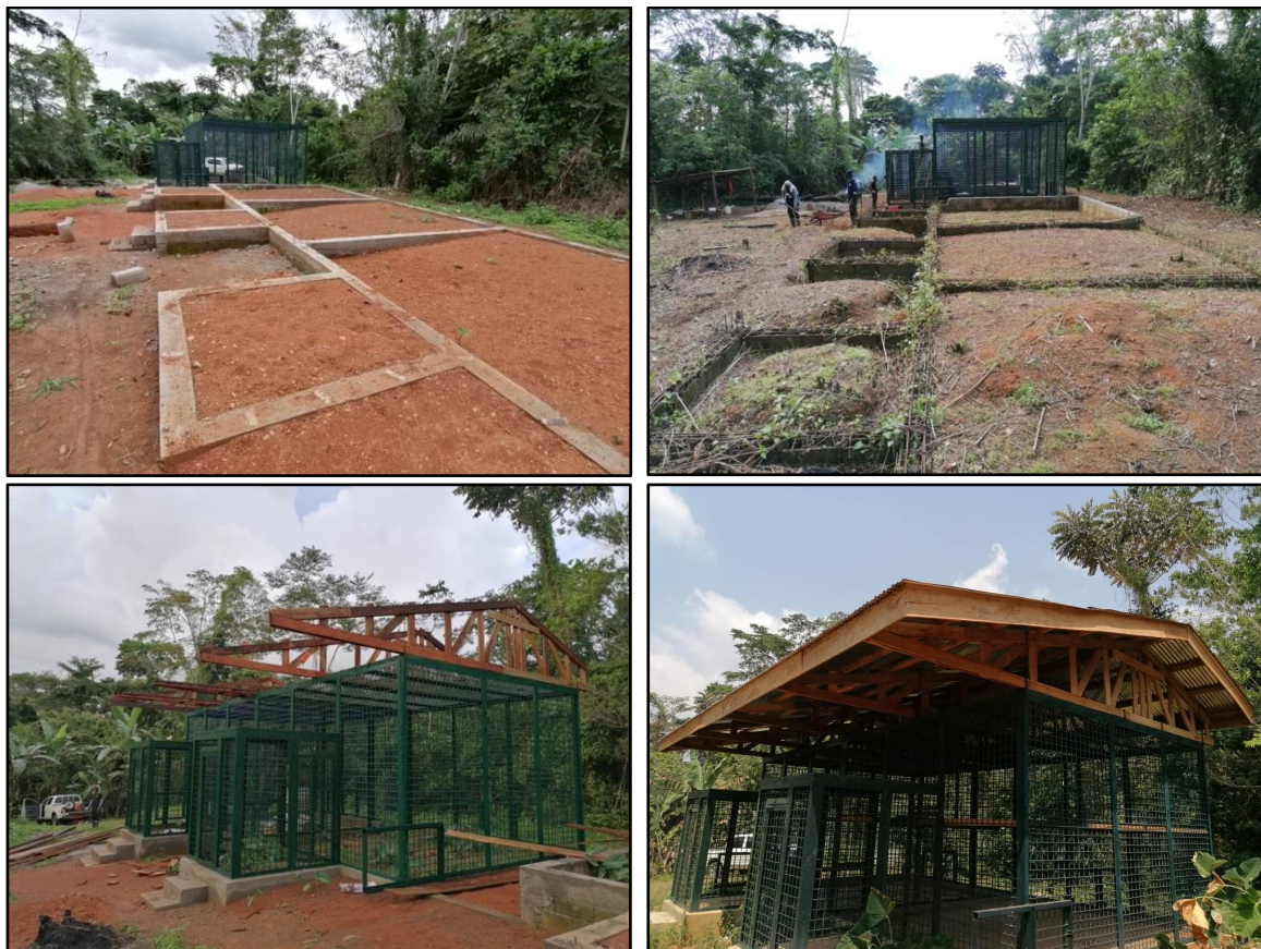
Photos showing the progress of the satellite cages of the high security chimpanzee enclosure.
