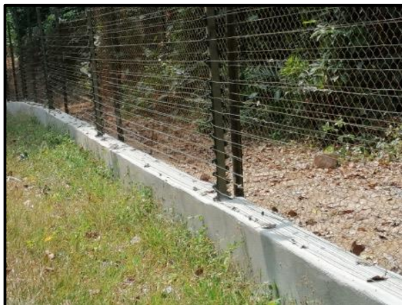
section of the new foundation at the chimpanzee enclosure
