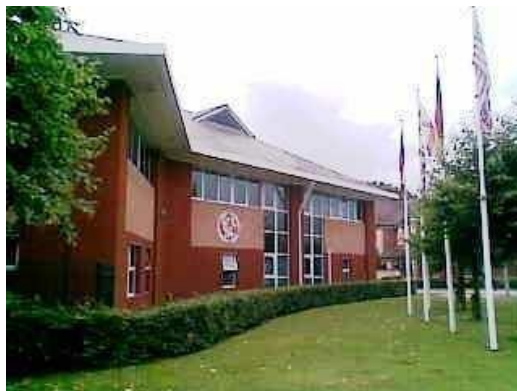
MVS Headquarters International Business Centre Warrington
