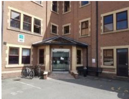
The Main entrance -Dallam Court
