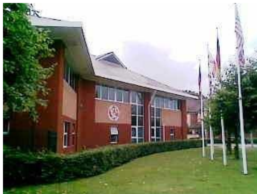
MVS Headquarters International Business Centre Warrington
