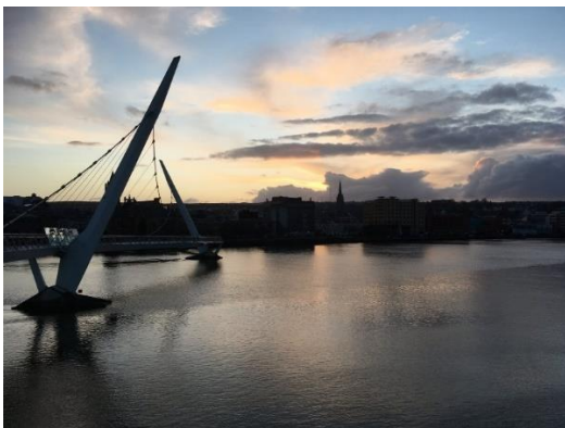
The Peace Bridge – Derry/Londonderry
