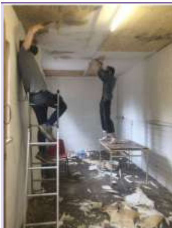
Ro & Aiden: stripping Camp Store ceiling for refurbishment
