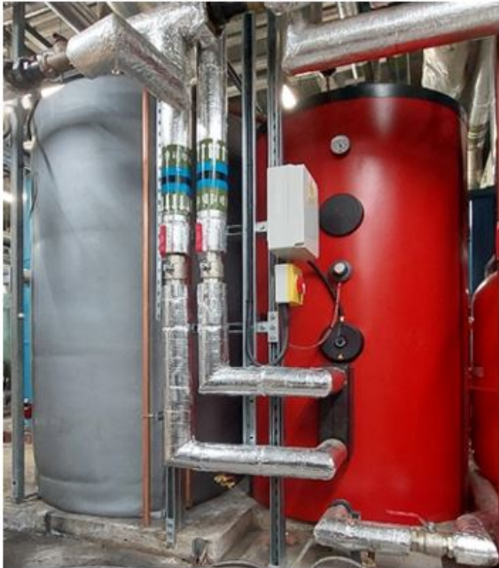
New calorifier & pre-heat vessels
