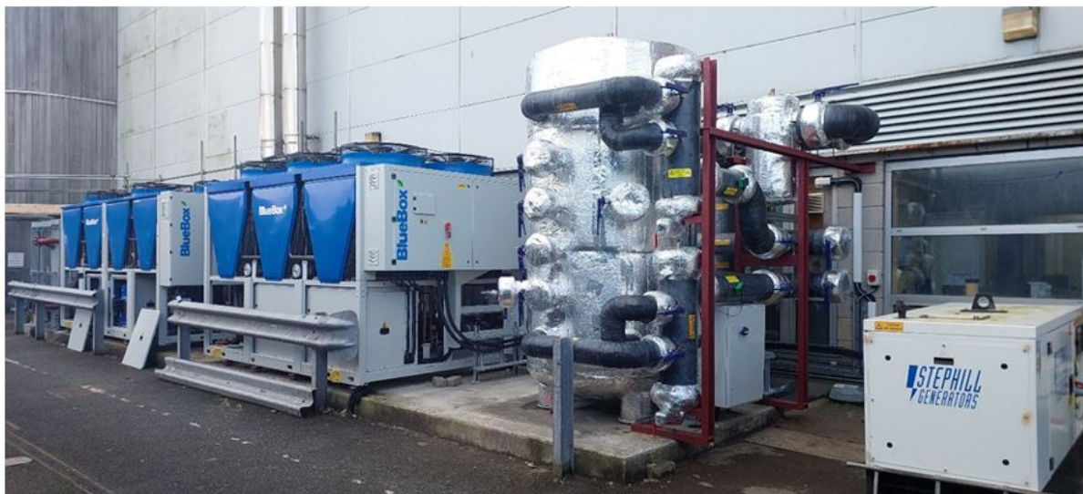
Newly installed chiller, heat pump, and associated thermal vessels
