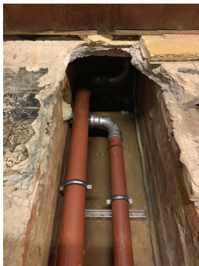
Pipework at Abington – before and after
