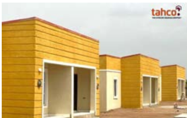
FIGURE 9: THE AFFORDABLE HOUSING COMPANY (TAHC), KUJE
